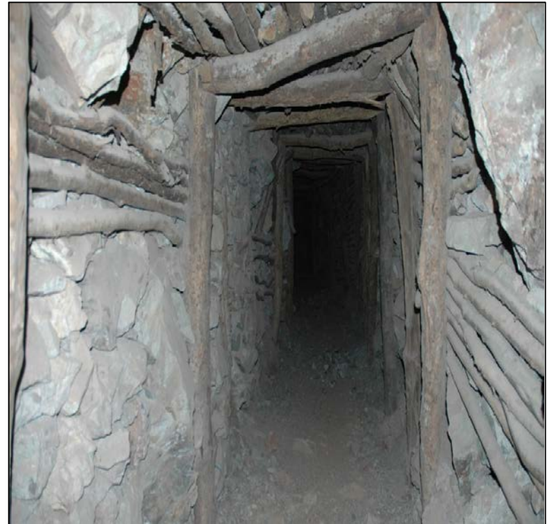
Bell Vista Tunnel – La Raya System
