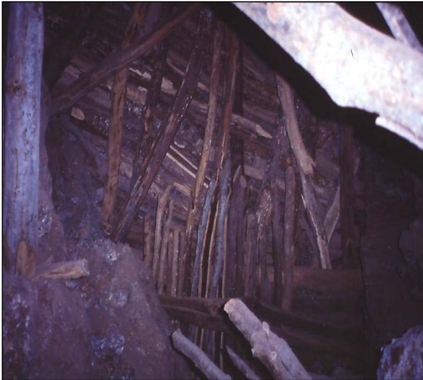
Socavon Intermedio –timber wall holding up backfill
